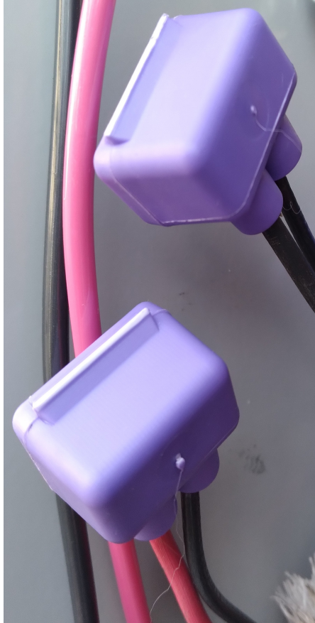
AlumiConn 15 Amp circuit 14 AWG wire
