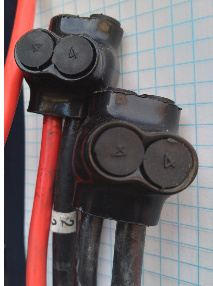
Morris or Polaris, 60 Amp circuit 4 AWG Aluminum – 6 AWG Copper
