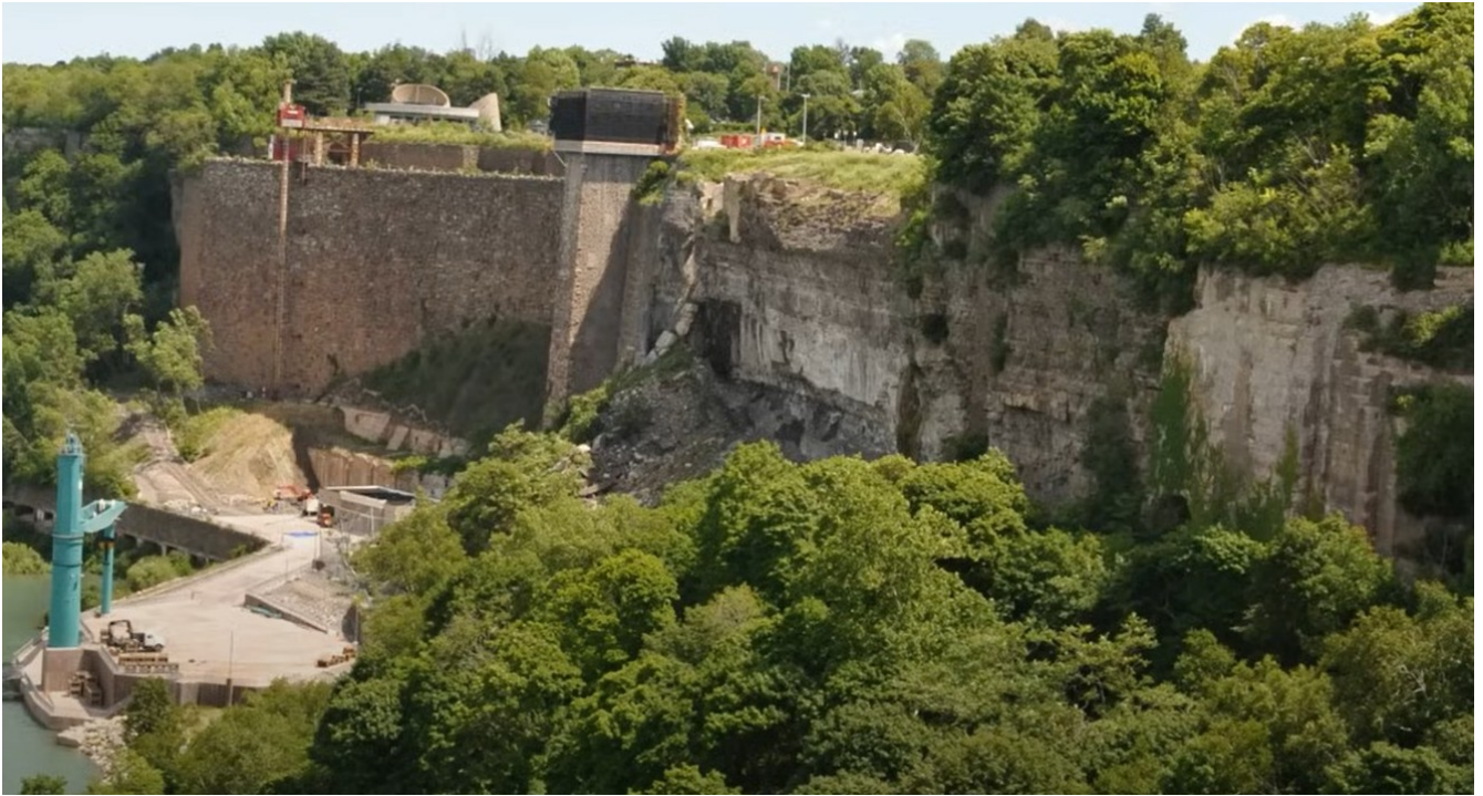
Schoellkopf Power Plant: 1956 Collapse & Ruins Today
