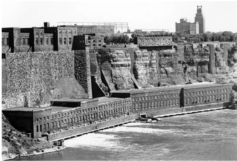
Schoellkopf Power Plant, 1924 – 1956 3-A (left), elevator shaft, 3-B (center), 3-C (right)
